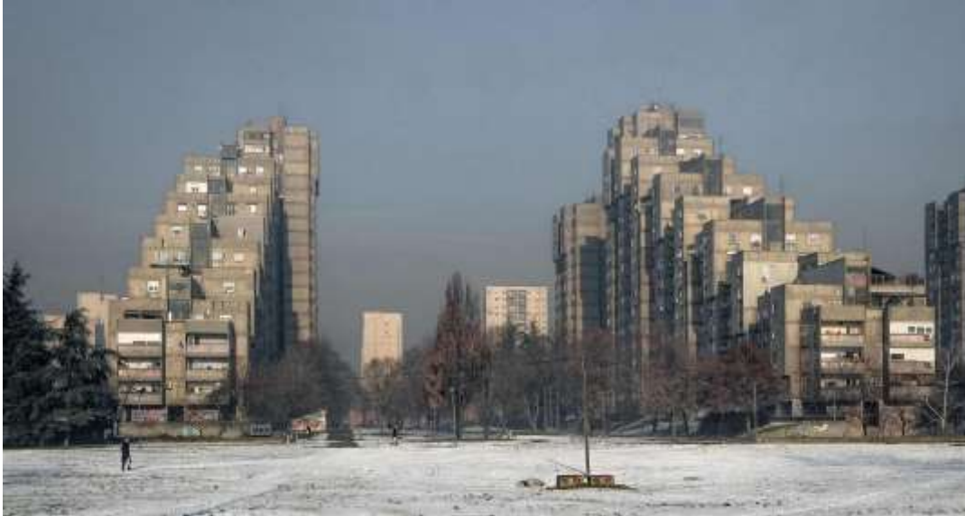
Photo 4. Blocks 61-64 (Officer blocks or Panonian Sailboats), Belgrade, Serbia, Built in sistem RAD-BALENCY - between 1974-80, Architect Milan Miodragovic. Urban design Josip Svoboda.
